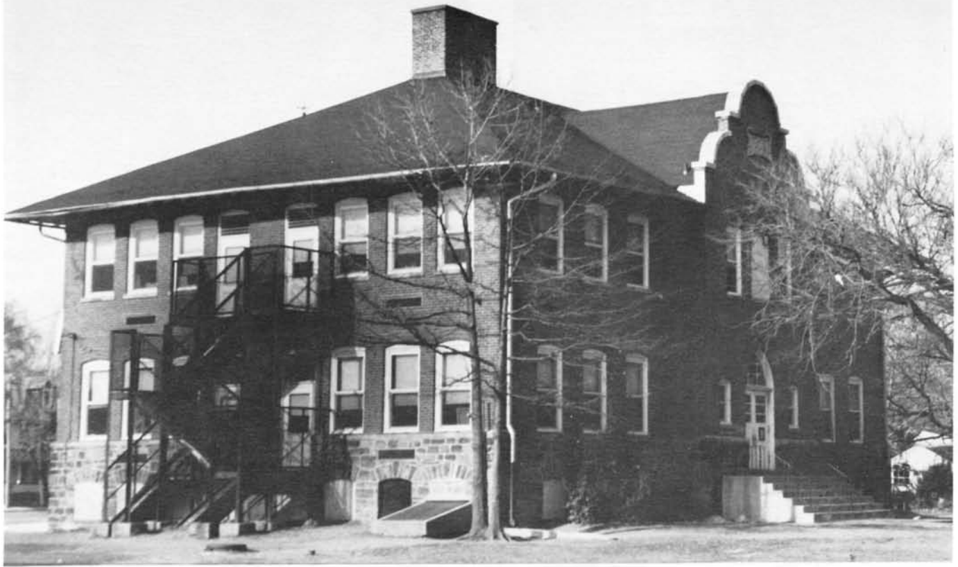
THE HICKORY STREET School was built in 1902. Delanco's second school was a two-story brick build-
