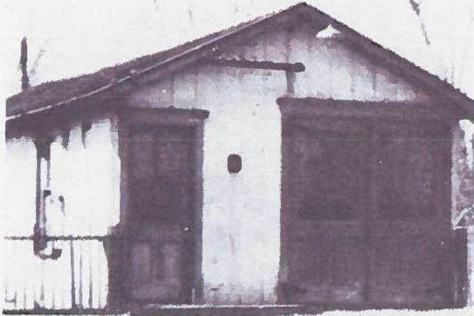
THE ORIGINAL firehouse in Delanco was this one-story structure shown on Union Avenue, where it had been moved from an earlier location on Ash Street.
