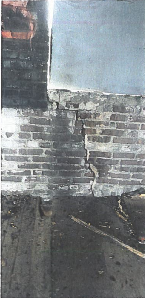
Exterior brick wall failure
