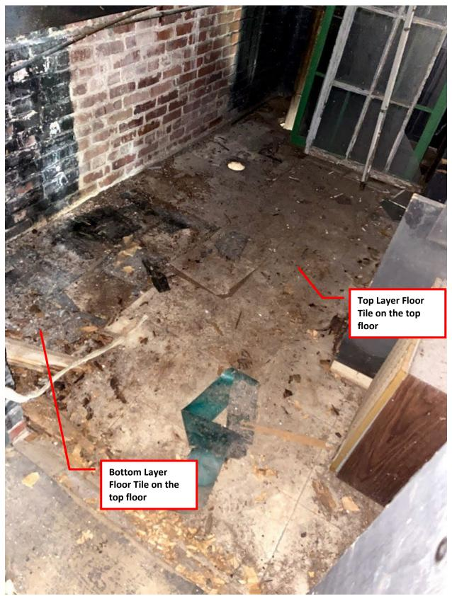
Figure 1: ACM Floor Tiles in the Western room on the top floor
